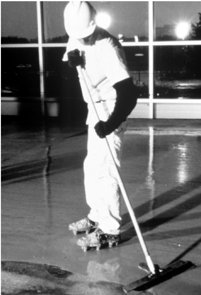
Figure 13. Self-leveling toppings can be used to restore the floor surface on an otherwise sound slab. Underlayments usually require a floor covering material such as tile or carpet. (69682)
